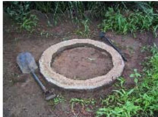
Add remainder of concrete mix, level off and ram flat with wooden float. Cover with plastic sheet and leave to cure for 10 days. Keep wet at all times. Then move to location on level ground.
