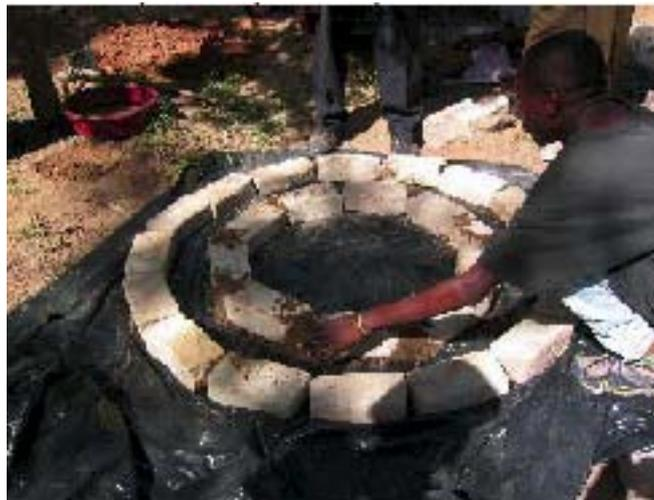
Once the brick mould has been made, make up the concrete mixture of 5 litres fresh cement with 30 litres good river sand. Mix the dry parts thoroughly first then mix with about 3 litres fresh water. Mix thoroughly again. Add half of this mixture to the mould. Then take a length of 3 – 4mm wire and place above the concrete mix about half way between the inner and outer bricks.
