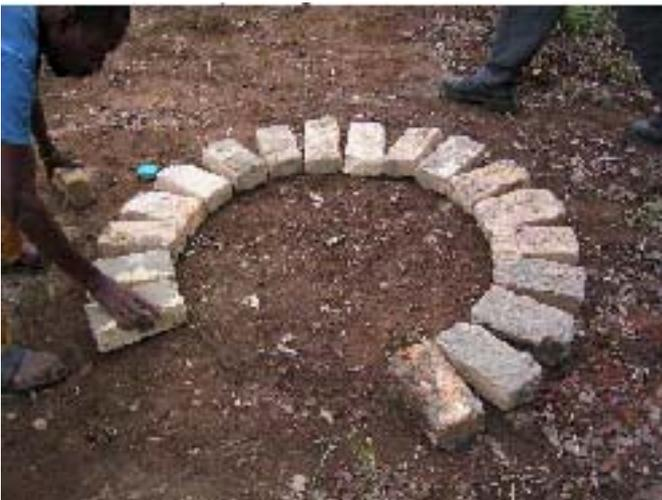
Now make up some ant hill mortar (Ivhu re pa churi) by breaking up ant hill soil and mixing with water. Using a trowel add the anthill mortar between and above the bricks.
