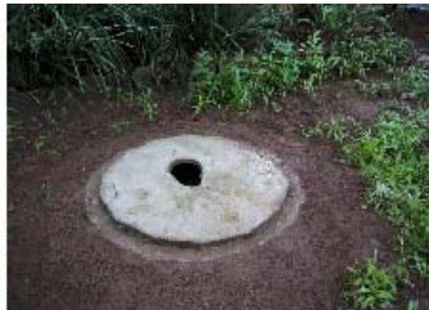
Dig down hole within the ring beam to at least 1 metre below surface. Place soil around ring beam and ram in place hard. Add leaves to pit base. Lay anthill mortar or weak cement on ring beam and place slab on top. Bed in and level the slab. The structure can now be built around the slab.
