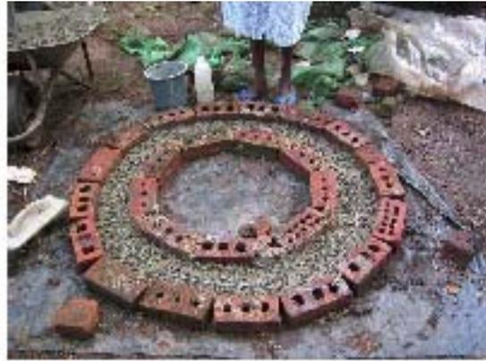
Fill in spaces between inner circle of brick mould with wet sand. Make the 6:1 mix of clean river sand and fresh cement. Add half the mix, level off and then add the circle of 3 – 4mm wire.
