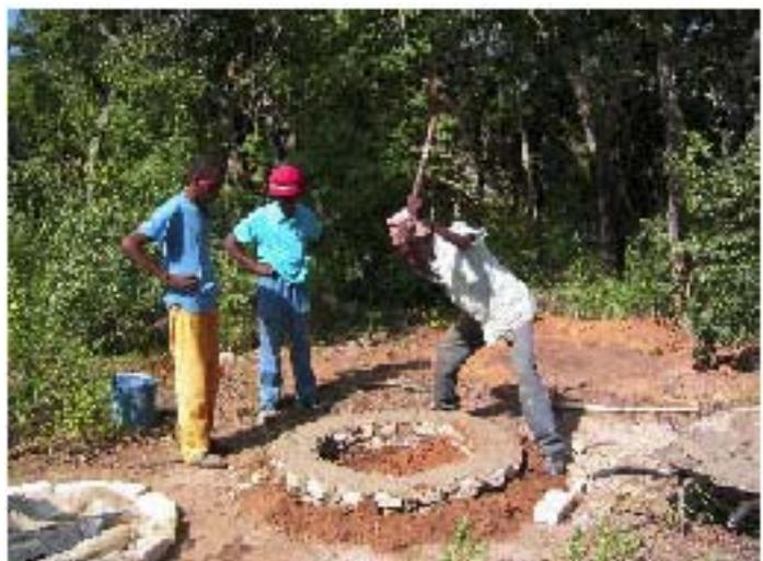
This ring beam and soil helps to raise the toilet above ground level and stops rain getting into the pit. The ring beam and surrounding soil helps to make the toilet stronger.
