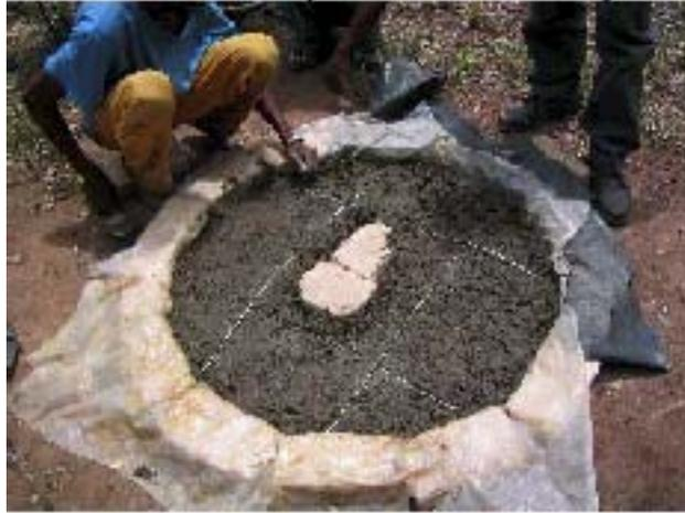
Add 4 reinforcing wires each 3 to 4mm in diameter and 90cm long in a square shape around the squat hole. Then add the rest of the concrete mixture. Spread out evenly.
