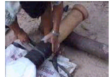
a pipe is tied with rubber strings The picture is from a biodifester and this does not have a "T"
