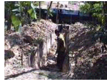
the trench is dug
