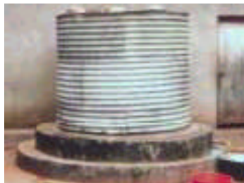
corrugated iron tank
