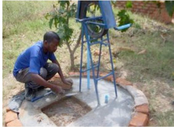
Figure 6: *Mounting the rope pump on concrete*
