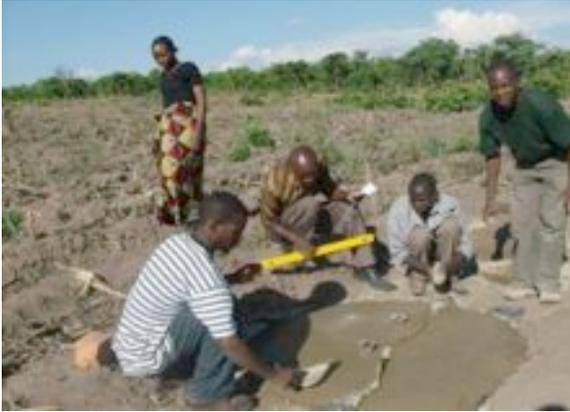
Figure 5: *Preparing concrete top-lid for the rope*
