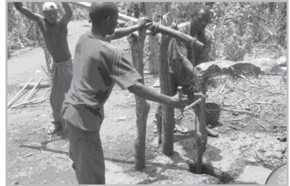
*Rota-sludge drilling in Northern Mozambique: 15-20 m in 3-4 days*
