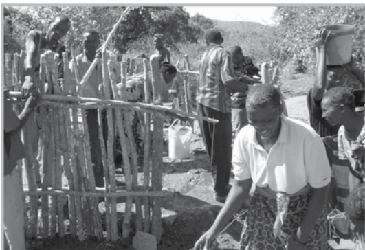
Building a pole fence to protect the water point
