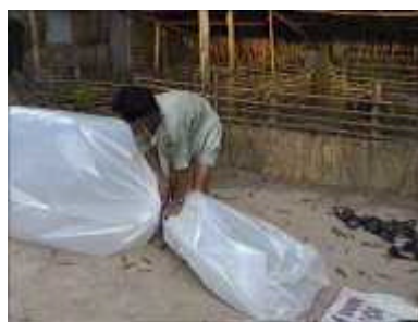
Photo 7. Tying the tube but leaving enough plastic to insert the outlet pipe
