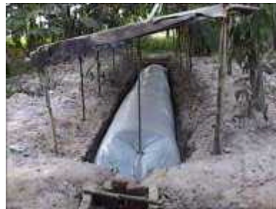
Photo 19. Roofing can protect the biodigester
