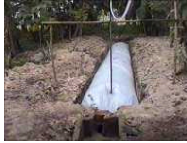
Photo 11. Connecting the PVC pipe to the gas outlet
