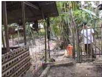
Photo 18. Fencing around the area where the biodigester is located
