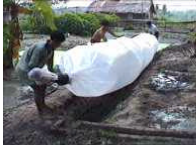
Photo 10. Placing the digester in the trench
