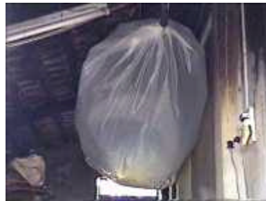
Photo 15. The reservoir bag full of biogas
