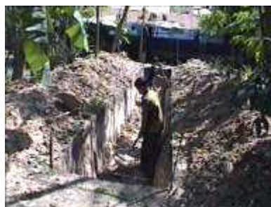
Photo 1. Excavating the soil
