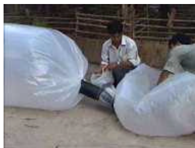
Photo 9. Forcing the air from the 3m tube to the main tube
