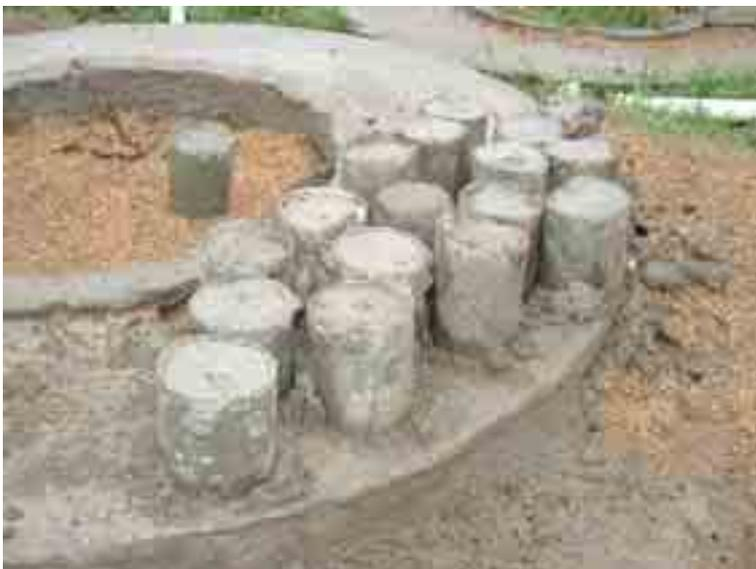
The bottle is cut to make a clean cut using a piece of rope (not nylon but natural fibres) tied around the bottle 15 cm from the bottom. The bottle is warmed over a candle or small fire in the area around the rope. Then the bottle is put into cold water and it will break along the line where the rope was. The bottom of the bottle is then filled with concrete, which is left to dry.
