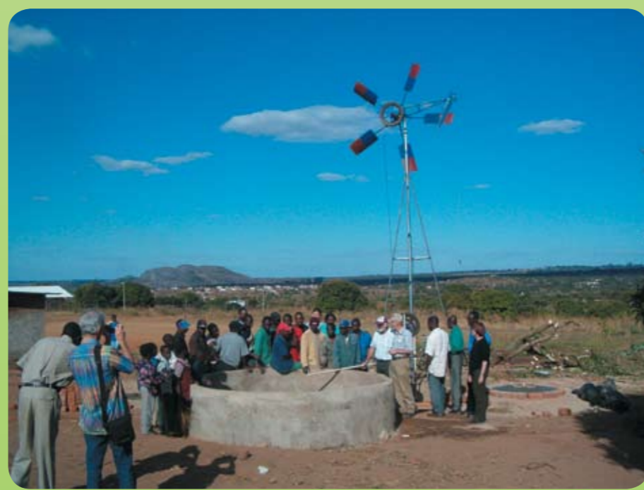
First windrope pump installed in Africa
