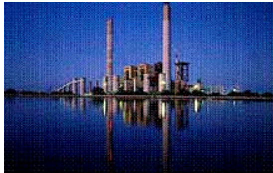
Figure 1: Matimba Power Station during construction
